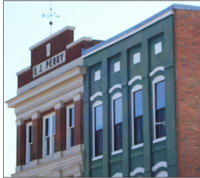
Upper windows are usually custom fit, large and have thick reveal due to the scale of facades.
