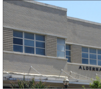
The custom designed upper windows above include architectural facade styles (note horizontal divided aluminum windows). Horizontal banded windows and cast concrete frames are important to the "International Style"
