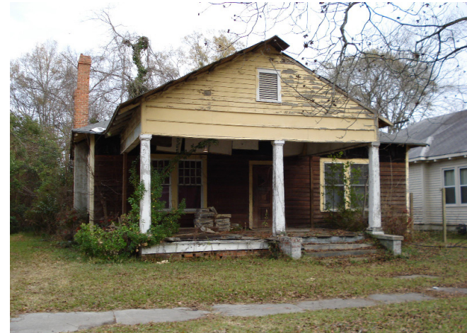
(Above) This is an example of a structure which, given more time in a vacant condition, may need to follow a "mothballing" routine. (Below) An illustrated concept of simple mothballing measures.
