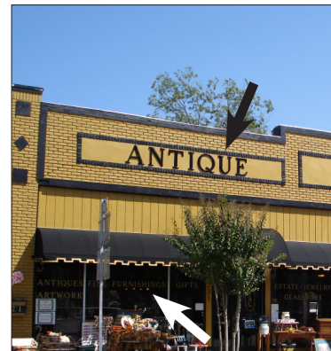
Keeping sign information simple and placed in traditional locations is key in the downtown commercial district where businesses are close together. Fitting simple, bold lettering within prescribed sign space is appropriate.
